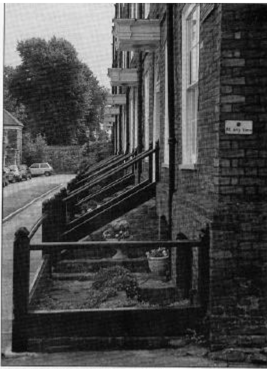
The railings that survived ( see overleaf ).
